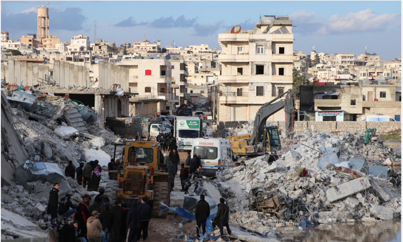
Thousands of buildings in Syria and Türkiye were flattened by the earthquakes, trapping people under the rubble.
